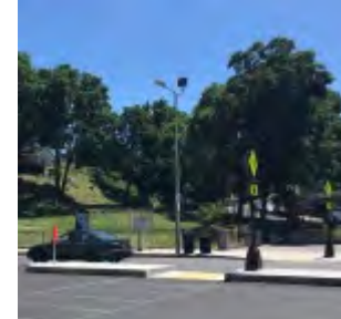
crosswalk, refuge island, rapid flash beacons
