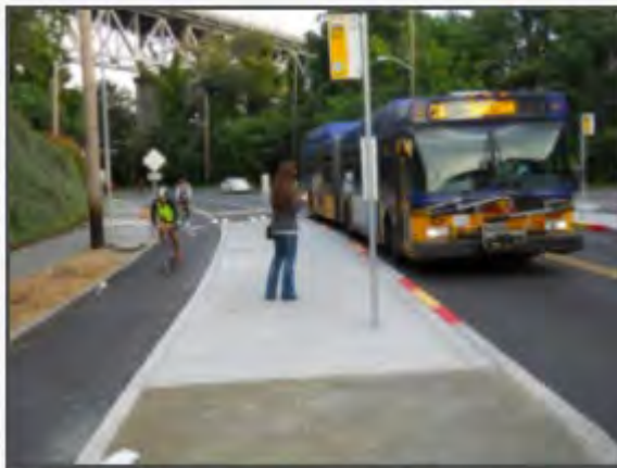
Bicycle lane placed between curb and transit stop platform, Seattle, Washington Source: Michael Hintze, Toole Design Group
