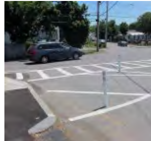
Crosswalk and curb extensions
