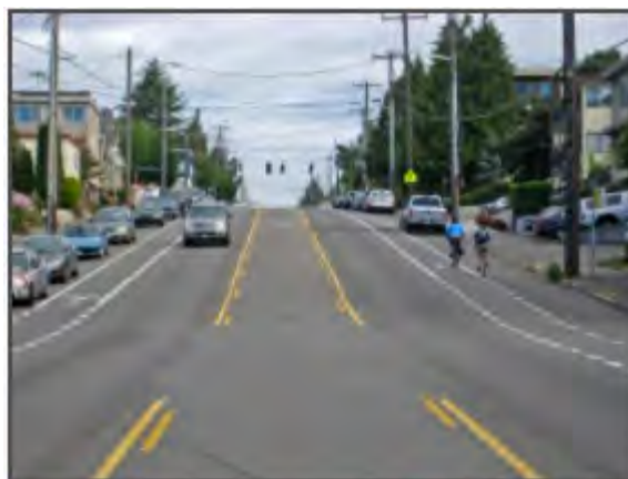
Lane diet (center lane narrowed) creates space to install bike lanes which also provides additional buffer for pedestrians on sidewalks. Seattle, Washington Source: Gina Coffman, Toole Design Group
